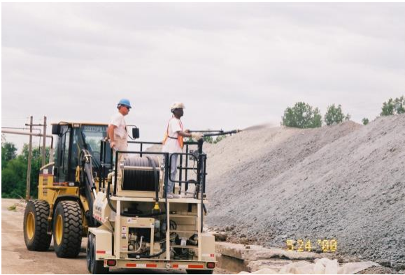
Applying ConCover 180 to the Contaminated Soils
