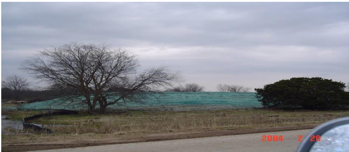
Final Restoration of Area M Landfill after Con Cover SW and seed application
