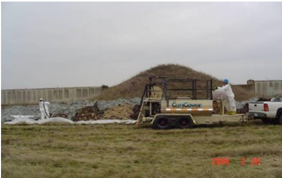
Applying ConCover 180 to PCB Contaminated Soils
